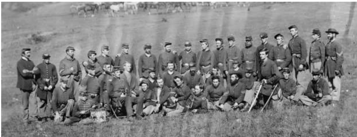
93 rd NY (AUG-NOV 1863) showing a mix of sack coats, Frock (dress) coats, Infantry Jackets, State Jackets, and musician Frocks. All enlisted (save for the sergeants) wearing forage caps.
